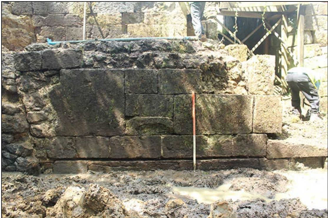
Figure 16 The south wing wall on the eastern side of the spillway
