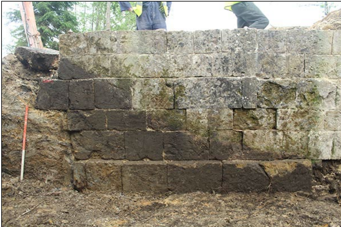
Figure 10 The upper step in the main east wall of the spillway at its southern end
