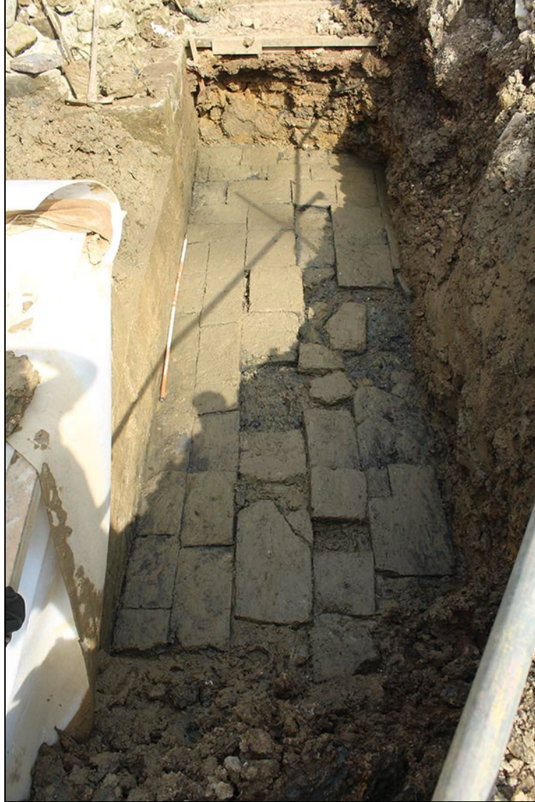
Figure 20 The stone apron to the east of the spillway, looking north
