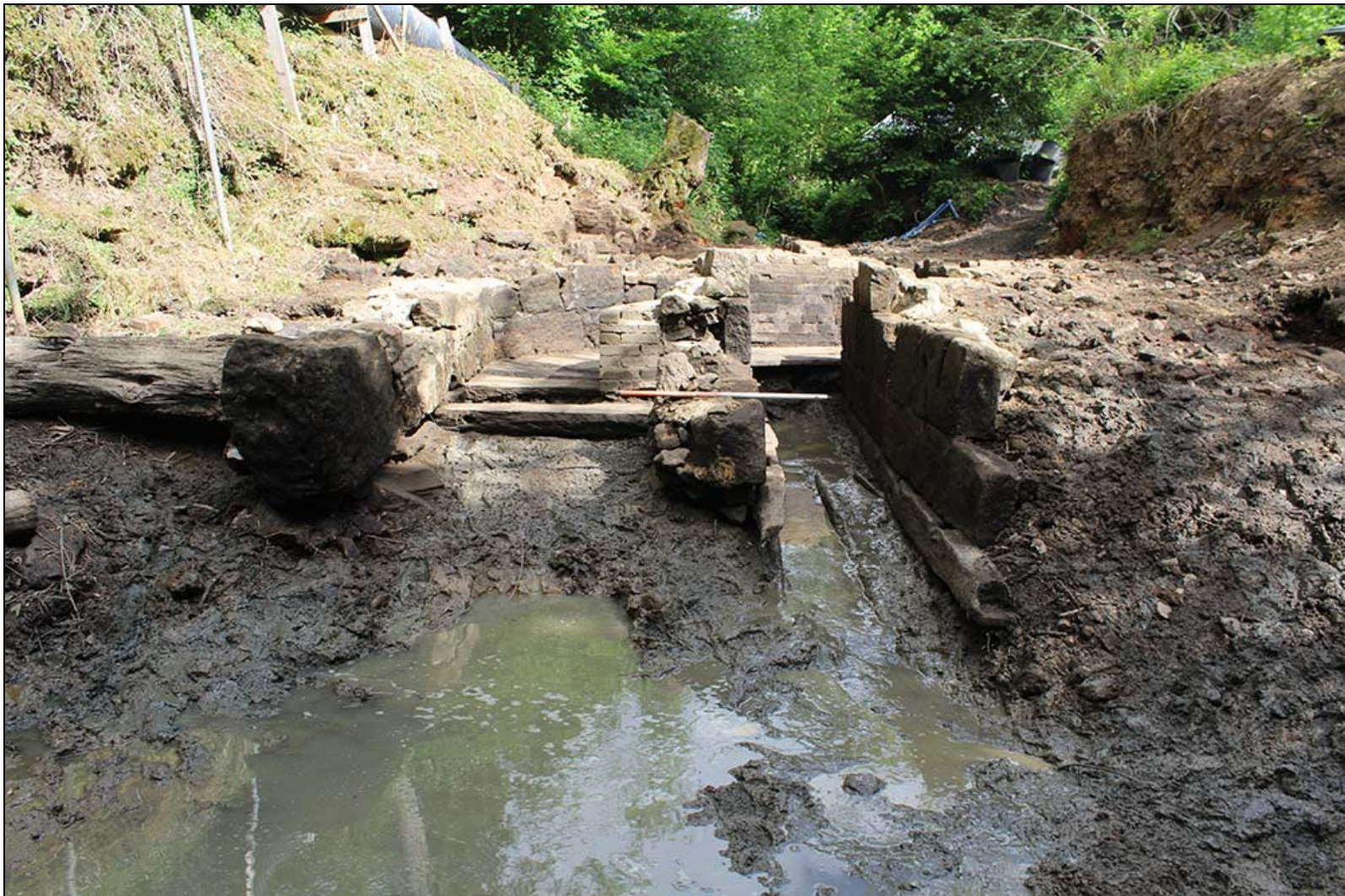
Figure 7 The entrance to the surviving wheelpits, looking south-east, showing the displacement of the outer walls, and the diminished central wall
