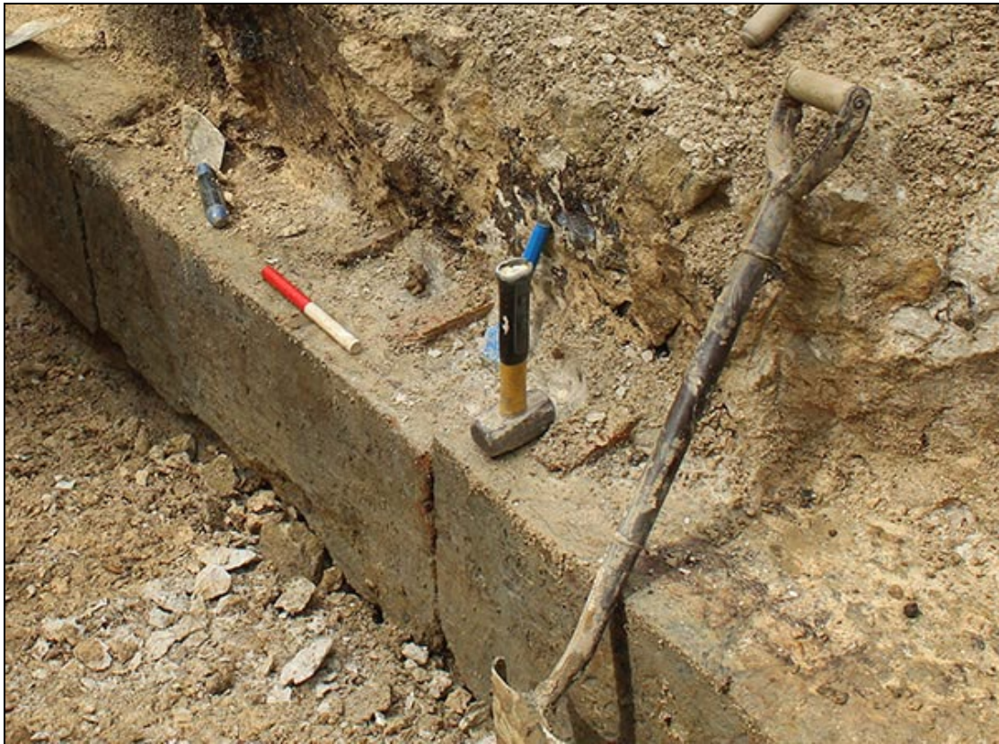
Figure 11 Three wooden wedges in the main east wall of the spillway
