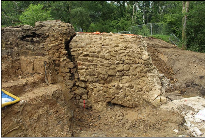
Figure 21 The exterior of the barrel vault, looking north
