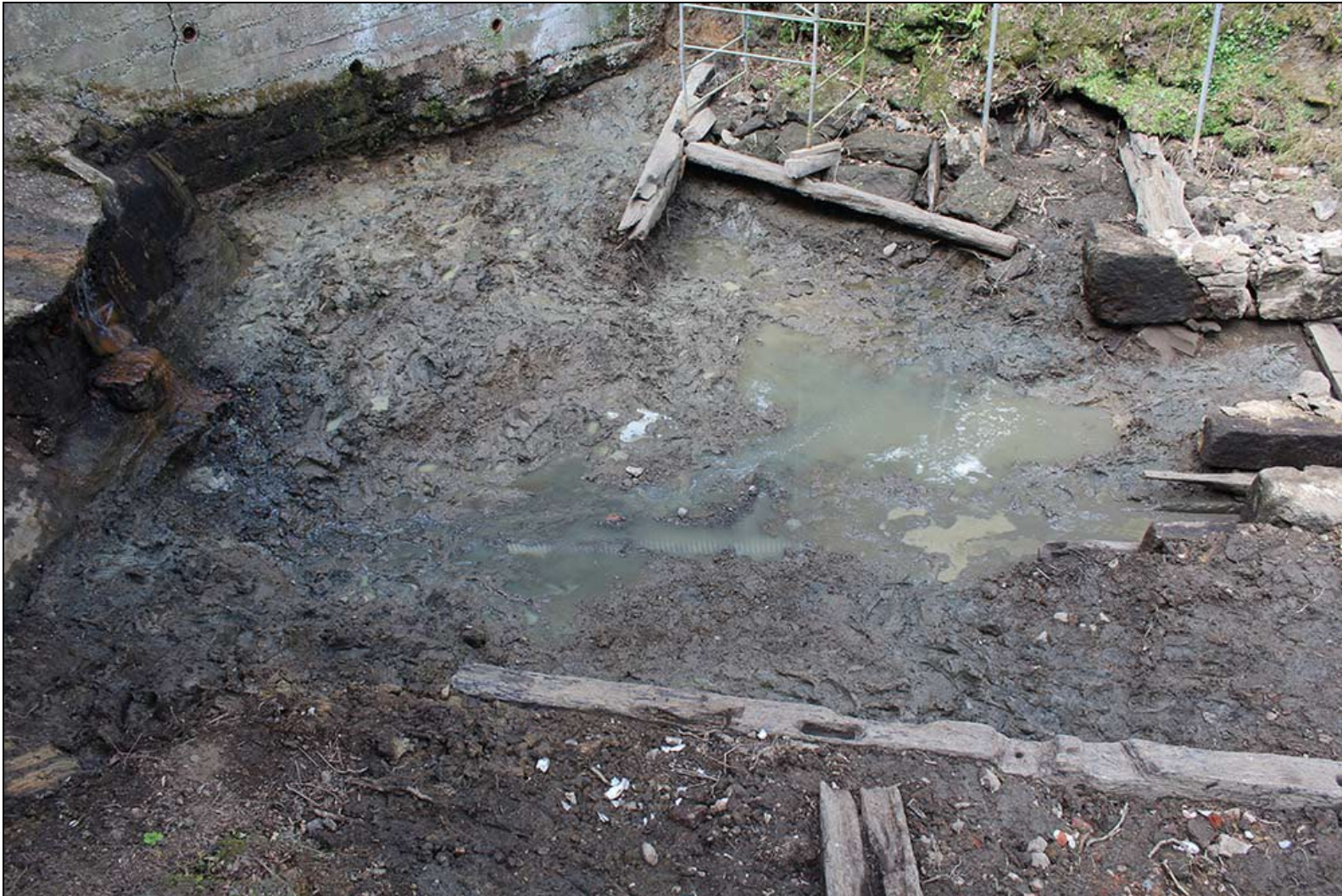
Figure 6 The wheelpit area looking north-east after removal of all the brick and stone debris onto the natural clay
