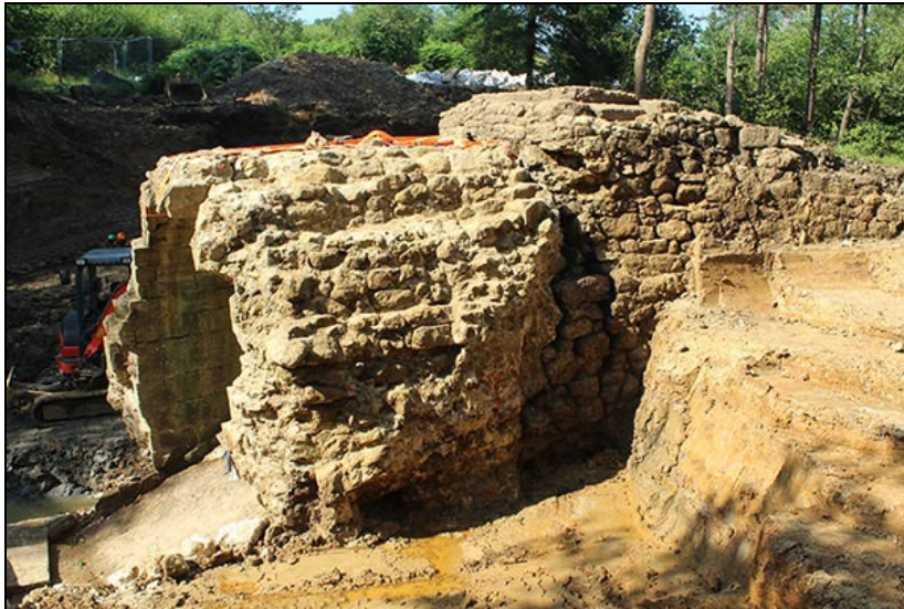
Figure 22 The exterior of the barrel vault, looking south-west
