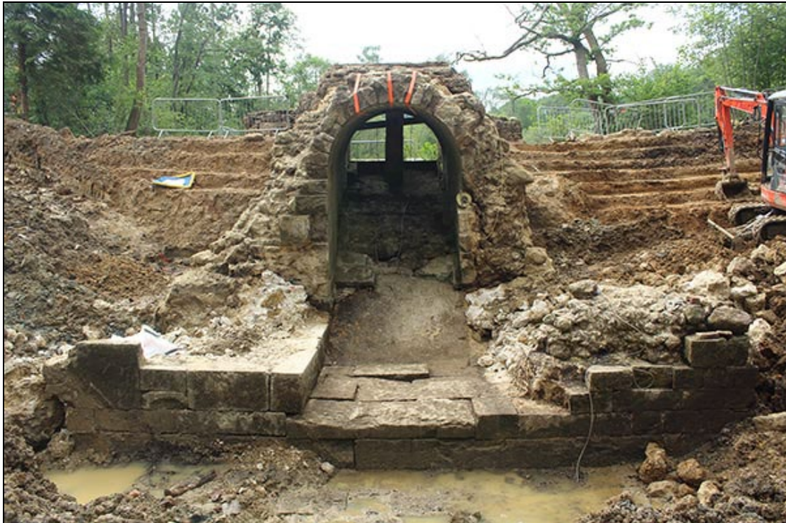
Figure 19 The spillway looking west, showing the remaining slabs at its base
