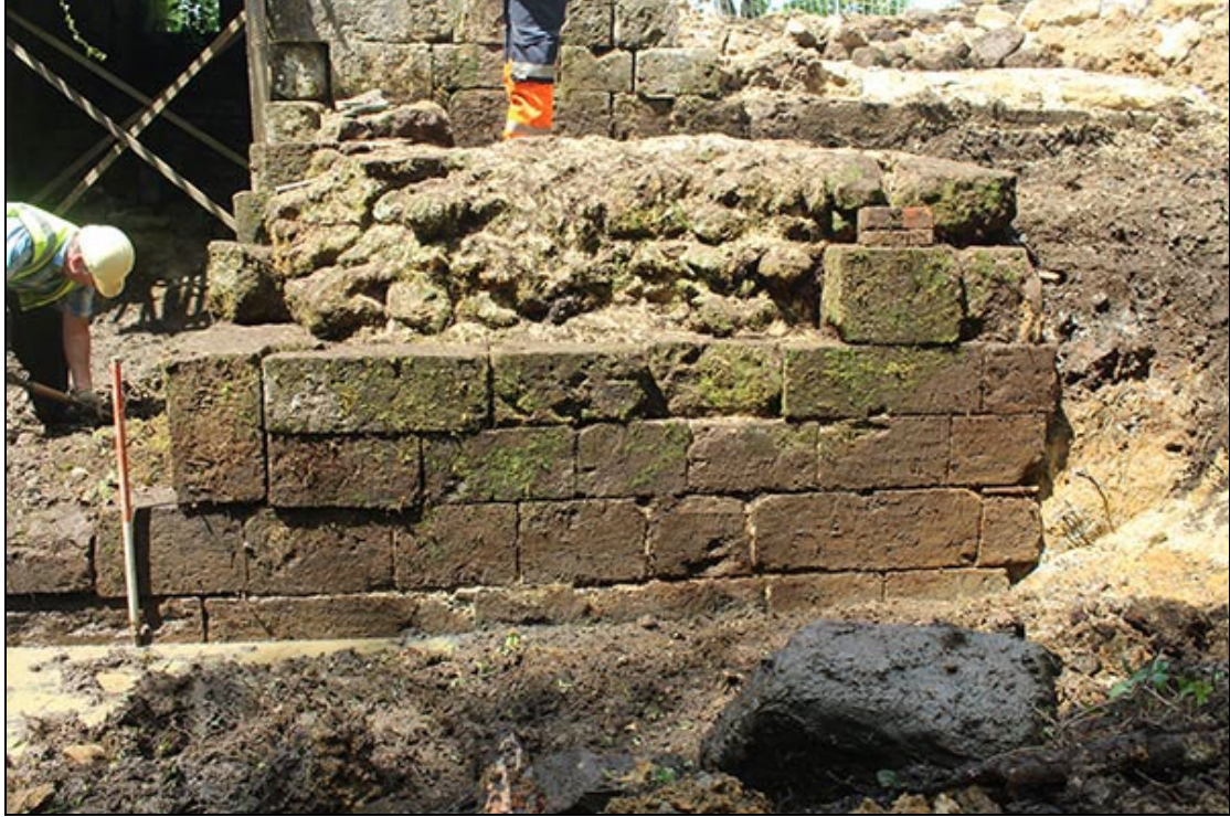
Figure 15 The north wing wall on the eastern side of the spillway
